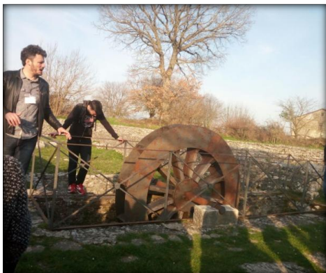
Figure 3-4 Of the original plant it remains a rectangular tank where it was placed a hydraulic wheel, moved by the raining water coming from the cistern set outside the walls. In the room at the back it was placed the milling system. The axis of the wheel passed through a horizontal opening and it milled a gear in a housing next to the wheel; upon it there were the millstones moved by a vertical axis.
